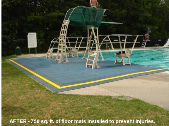
AFTER - 750 sq. ft. of floor mats installed to prevent injuries.
