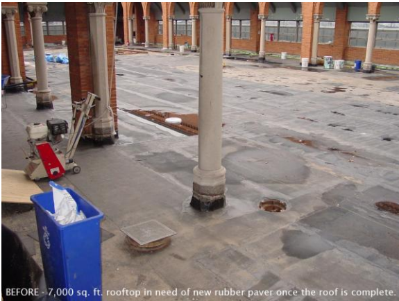
BEFORE - 7,000 sq. ft. rooftop in need of new rubber paver once the roof is complete.
