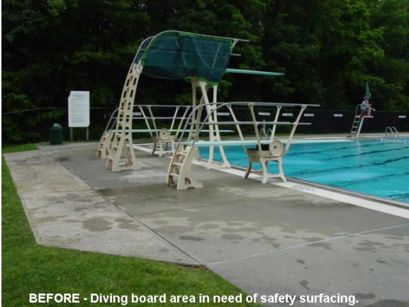
BEFORE - Diving board area in need of safety surfacing.
