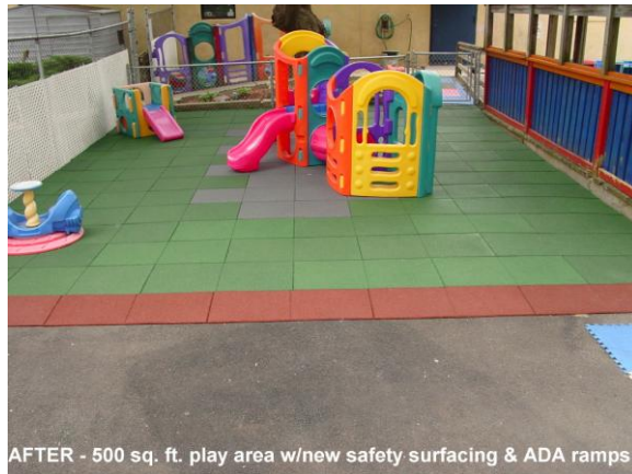
AFTER - 500 sq. ft. play area w/new safety surfacing & ADA ramps
