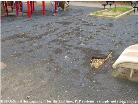
BEFORE - After capping it for the 2nd time, PIP systems is simply not strong enough
